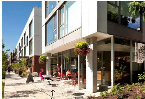
BEL ROY APARTMENTS WEINSTEIN AU Seattle, WA Transparent ground floor retail engages with the public realm and invites people in
