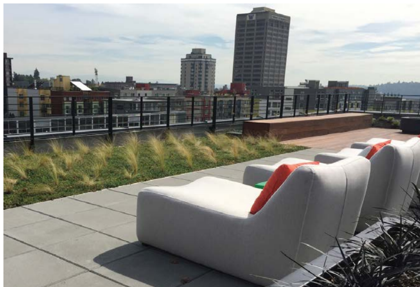
GREEN ROOF EDGE Seattle, WA
