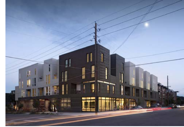
TEJON 35 MERIDIAN 105 ARCHITECTURE Denver, CO A minimal use of different exterior materials creates a timeless and maintenance-conscious palette
