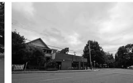
PHOTO OF EXISTING PROPERTY (ALONG BROOKLYN)
