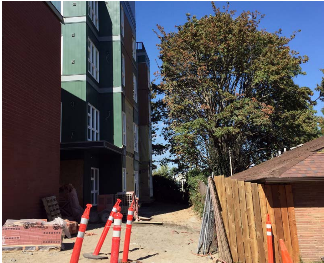
NEIGHBORING CONSTRUCTION FACING WEST
