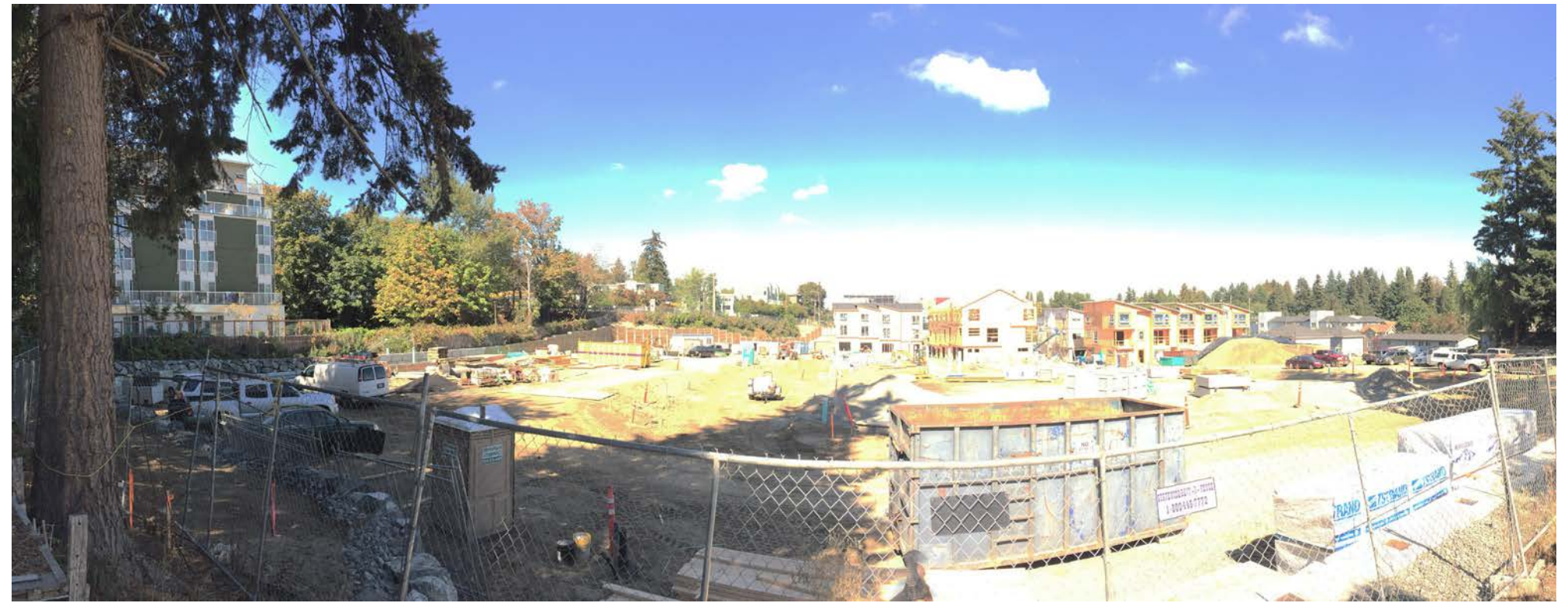
NEIGHBORING CONSTRUCTION FACING SOUTH
