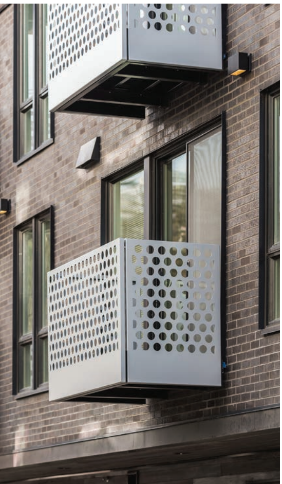
Perforated metal balconies
