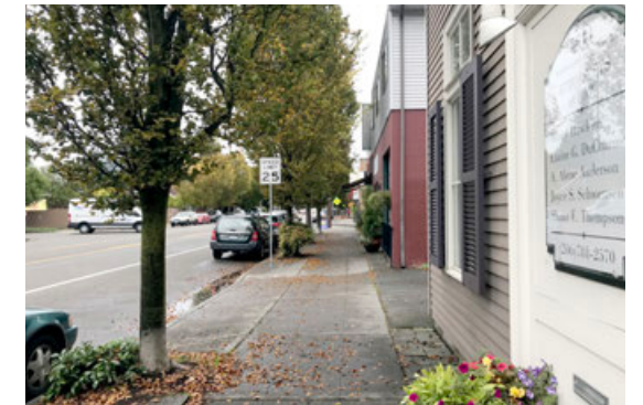
6. Greenwood Ave East - sidewalk condition
