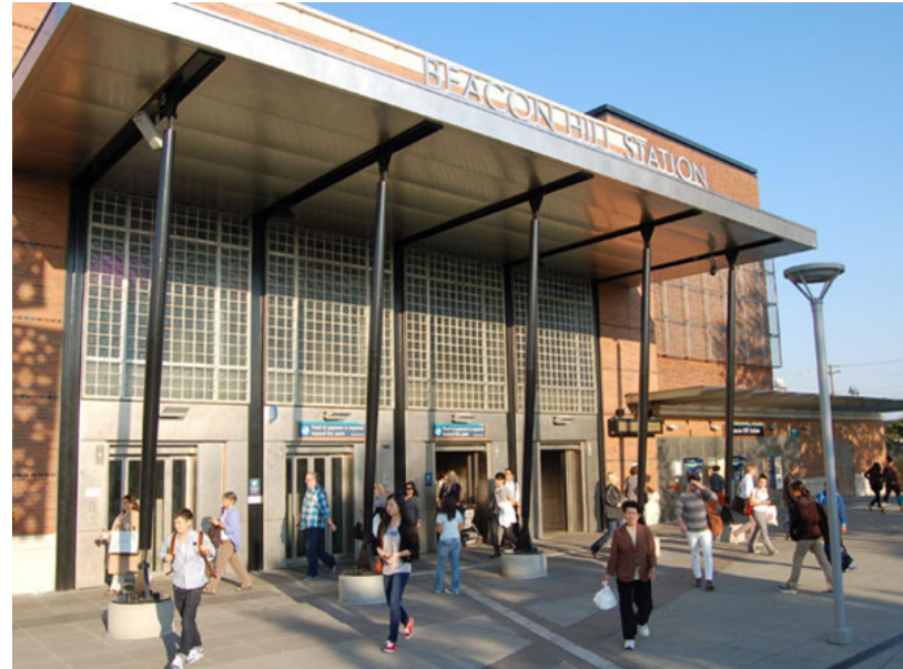
BEACON HILL STATION
