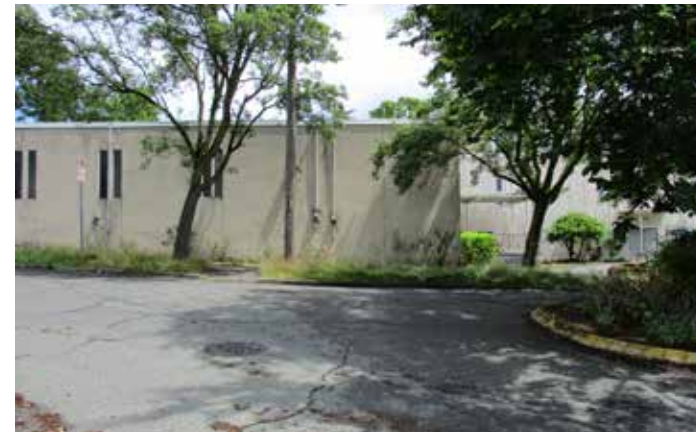
4 LOOKING AT PROJECT SITE FROM 28TH AVE S.
