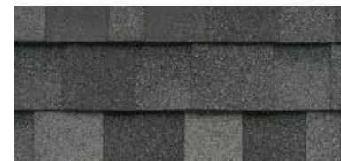
R1 Asphalt shingles Roof Gray
