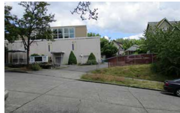
2 LOOKING AT PROJECT SITE FROM 28TH AVE S.
