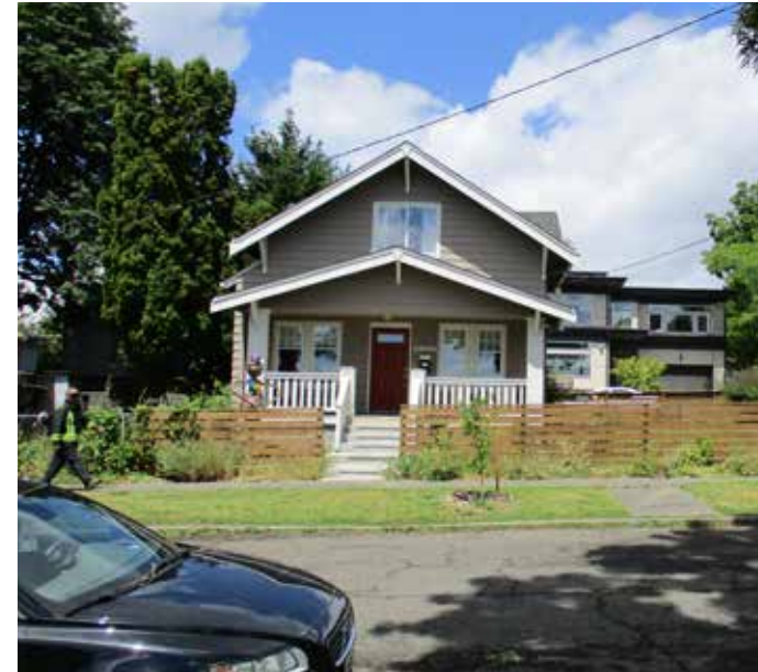
5 SINGLE FAMILY HOUSE ALONG S. DEARBORN ST.
