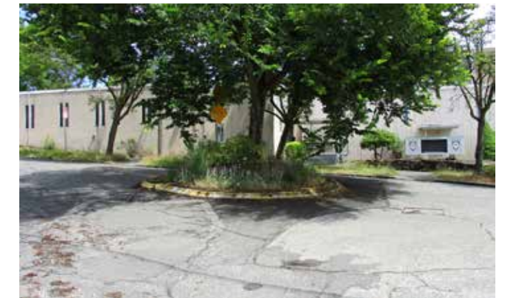
3 LOOKING AT PROJECT SITE FROM 28TH AVE S.
