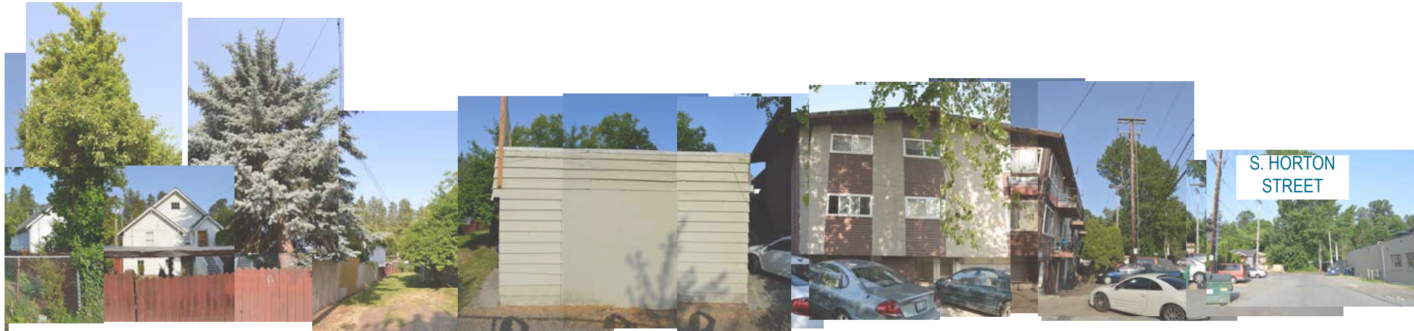
VIEW FROM ALLEY. LOOKING WEST
