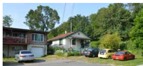
5. FROM SITE LOOKING SW
