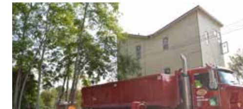
7. ONSITE LOOKING NE
