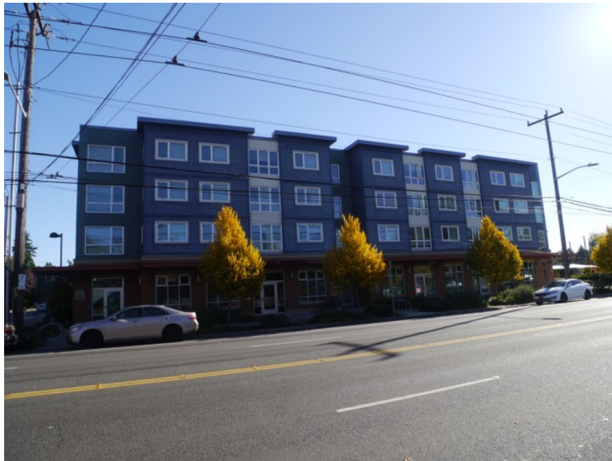
Rose St Apartments : Note façade modulation, roof lines, fiber cement cladding and simple geometry
