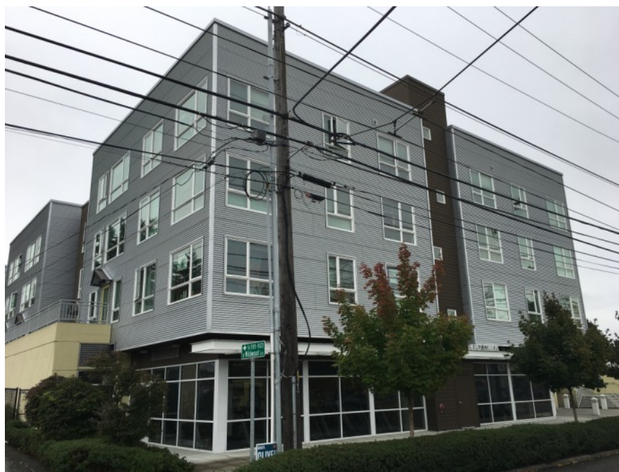
Emerald City Commons : Note façade modulation, roof lines, fiber cement cladding and simple geometry
