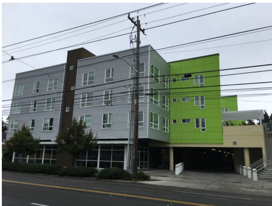
Emerald City Commons : Note façade modulation, roof lines, fiber cement cladding and simple geometry
