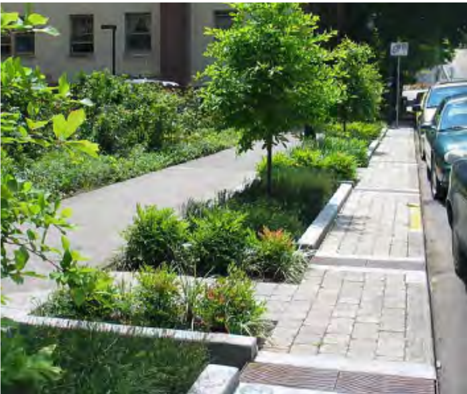
Bio-retention with weirs use the slope of the new street
