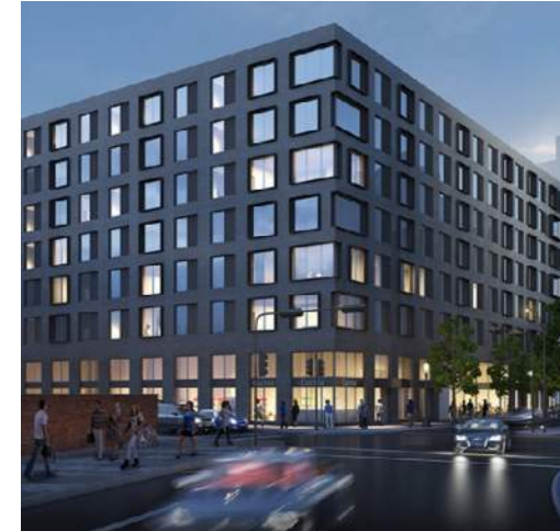
Facade Composition Windows provide texture
