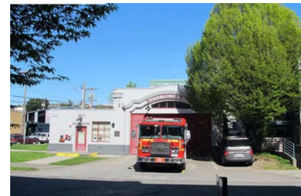
7 Fire station located on Oswego
