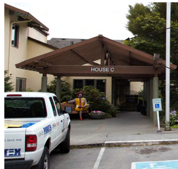
ASPHALT SHINGLE ROOFING
