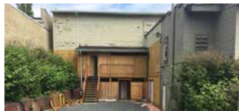
3. LOOKING E FROM ONSITE
