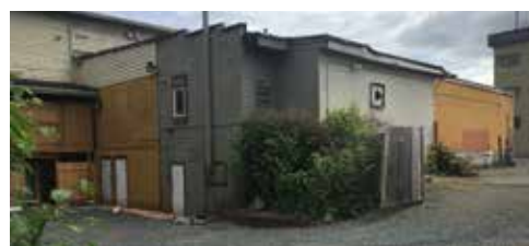
5. LOOKING SE FROM ONSITE
