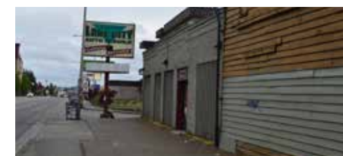
10. LOOKING S ALONG E PROP LINE
