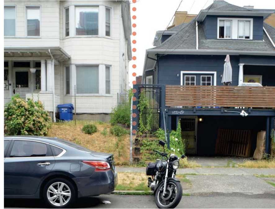
B North edge Note: elevated floor level of neighbor (white 3-story apartment building)
