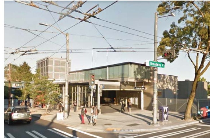
Capitol Hill Lightrail Station
