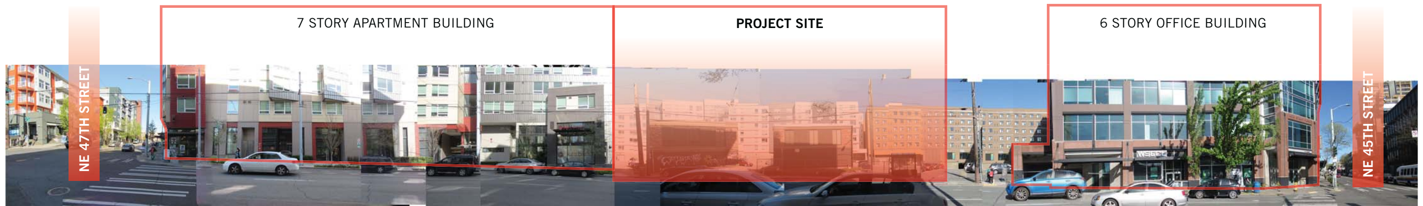
① 11TH AVE NE LOOKING EAST
