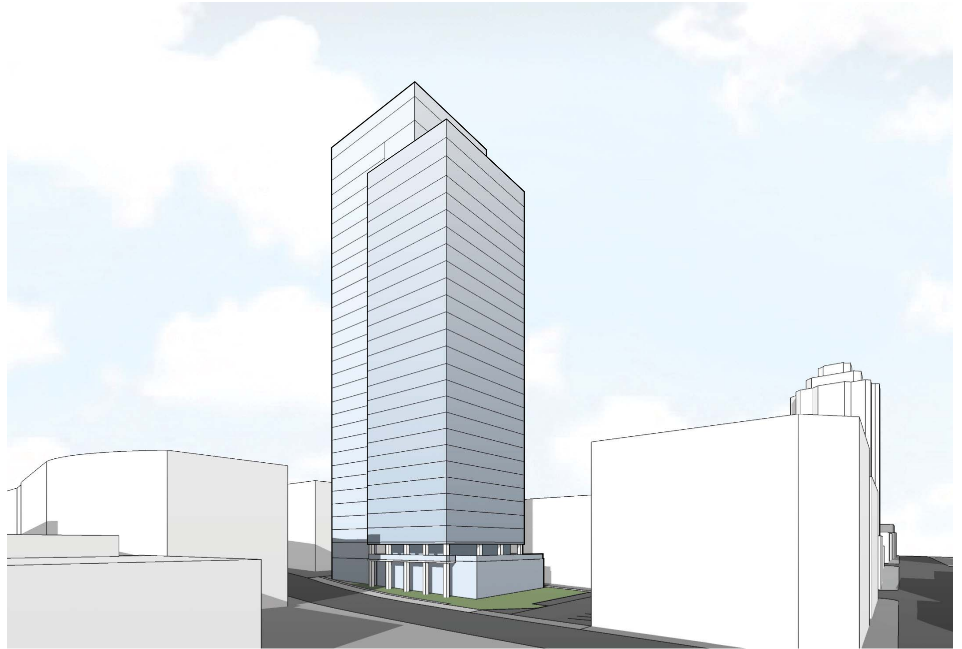
VIEW FROM SOUTHWEST
