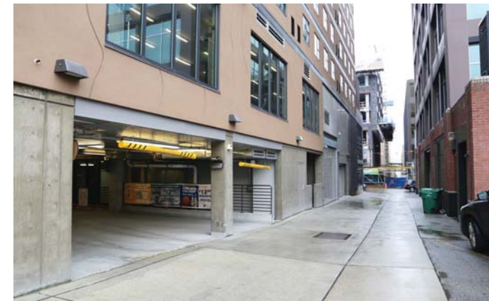
5 ALLEY LOOKING FROM THE NORTH
