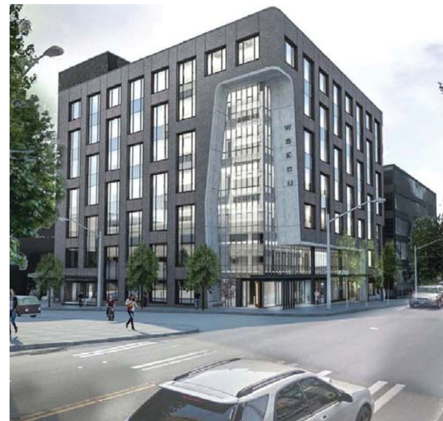
2 WSECU BUILDING UNDER CONSTRUCTION
