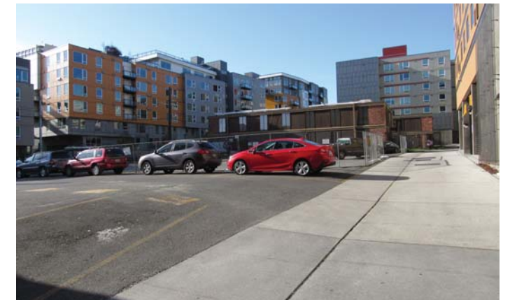
3 LOOKING FROM SE
