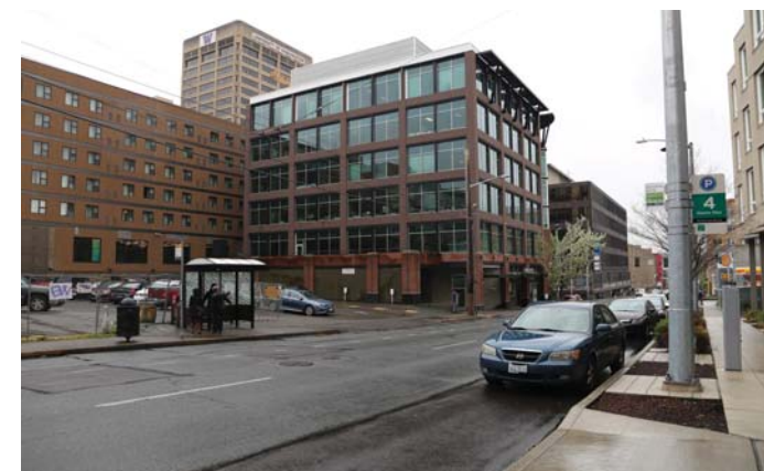
8 PROJECT SITE LOOKING FROM THE NW
