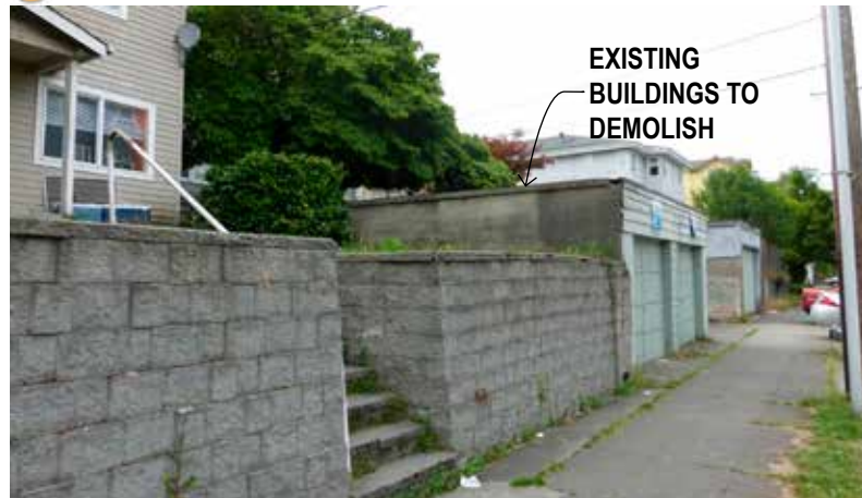
F NEIGHBOR BUILDING ON SOUTH FROM 20TH AVE NE
