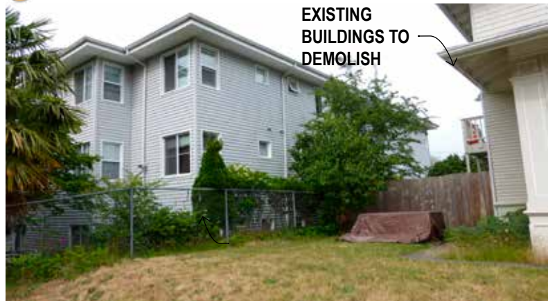
C NORTH PROPERTY & NEIGHBOR BUILDING ON NORTH
