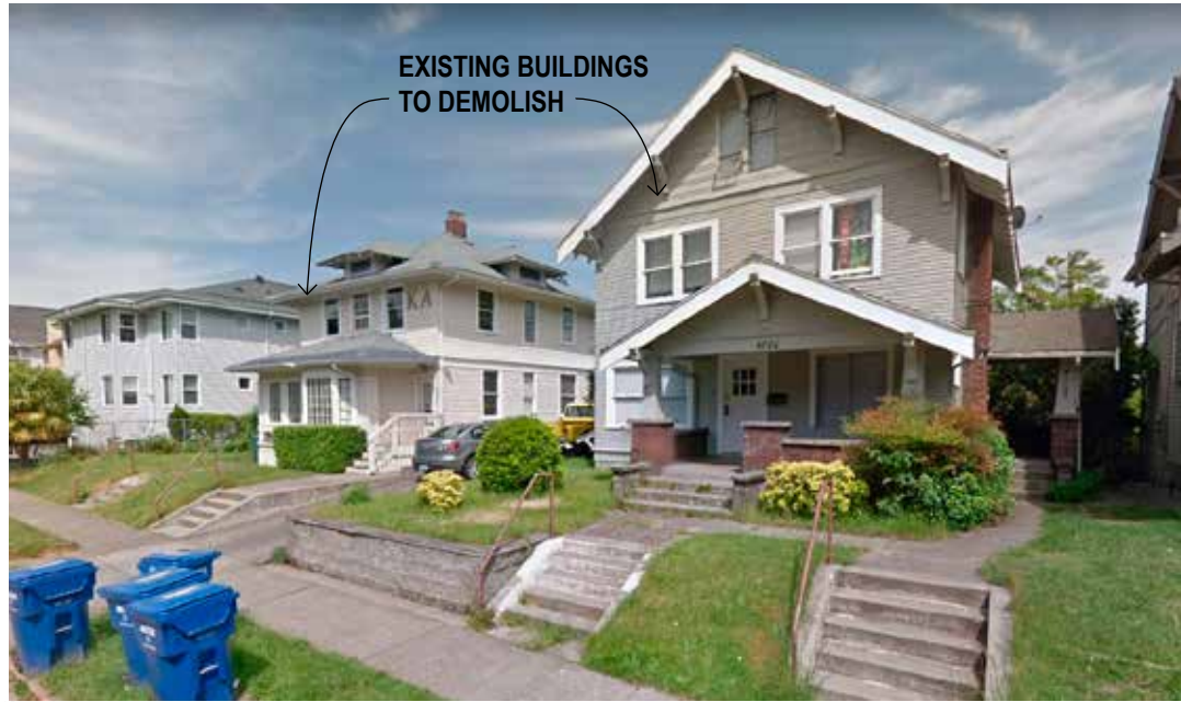
A 19TH AVE FRONTAGE FROM SOUTH
