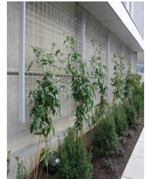
vertical green at alley
