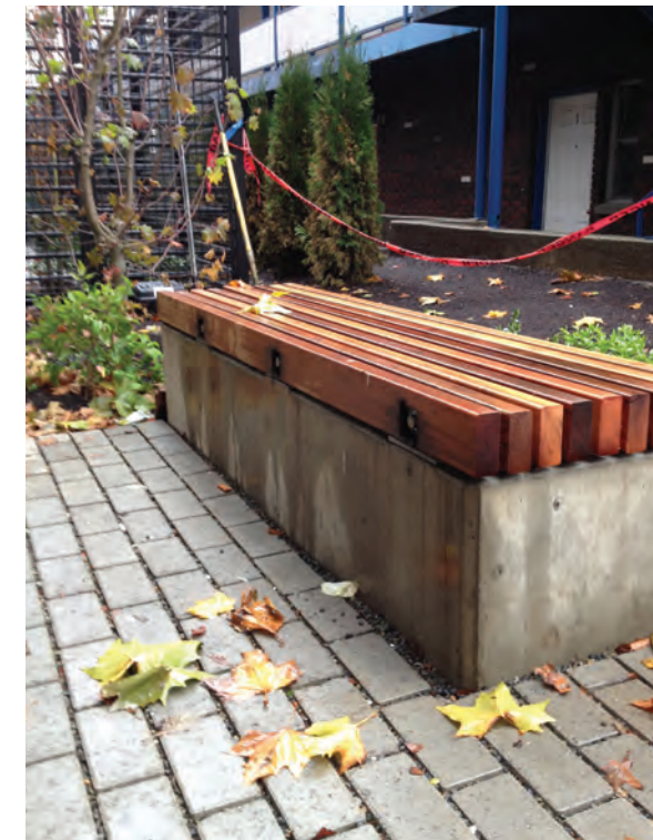
permeable pavers and seatwall
