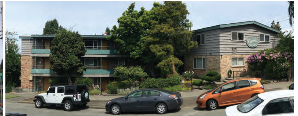
9 Kenwood Courts Apartments
