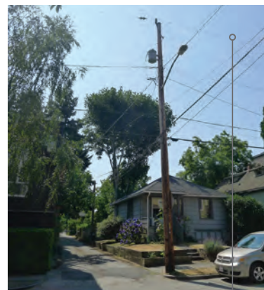
3 Electric pole 14' setback required from 26KV line along N 56th St
