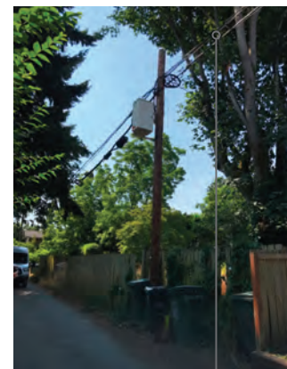
4 Comm pole Comm lines along alley to be undergrounded.
