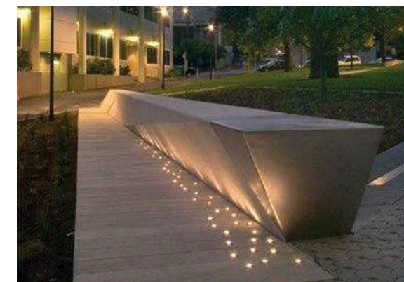
Feature Seating Pods with Lighting
