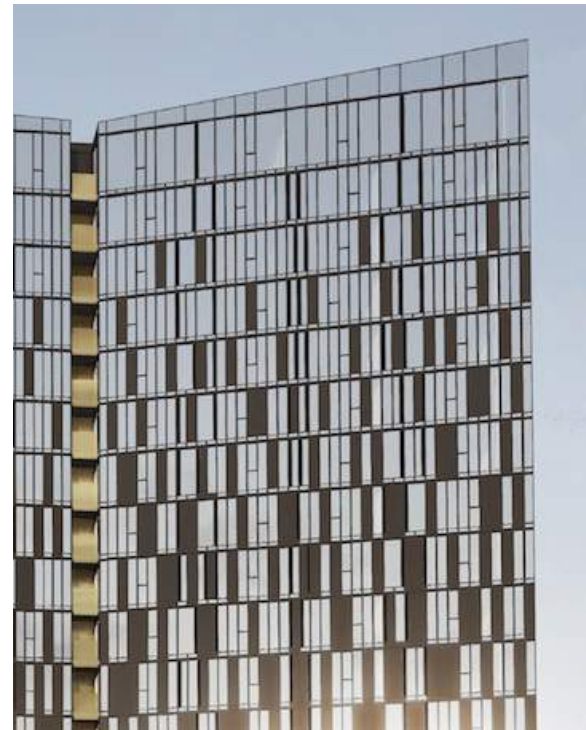
Metal panel character transitions from bottom to top of tower
