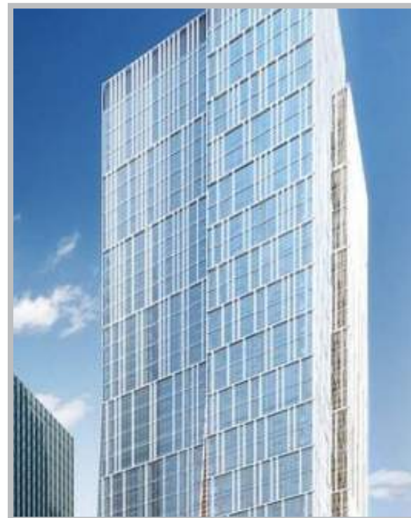
Vertically oriented metal panel and glass at tower
