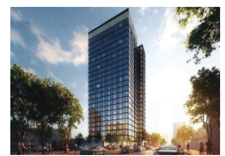
12 The M (Under Construction)
