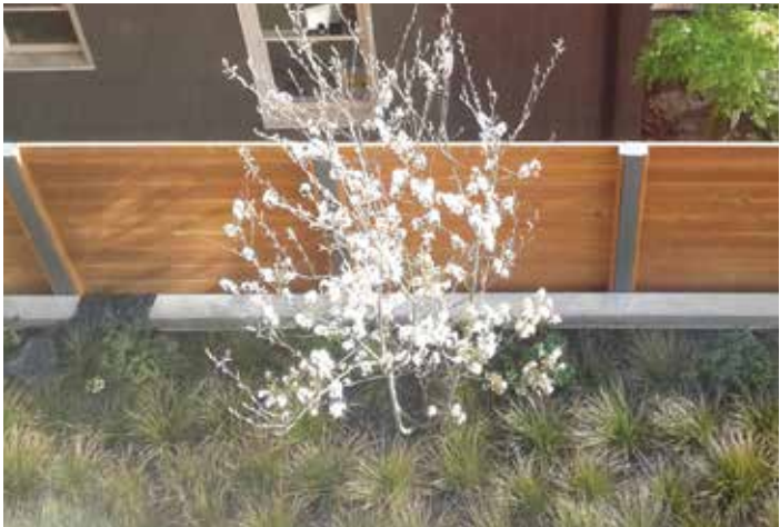
perimeter bioretention planter
