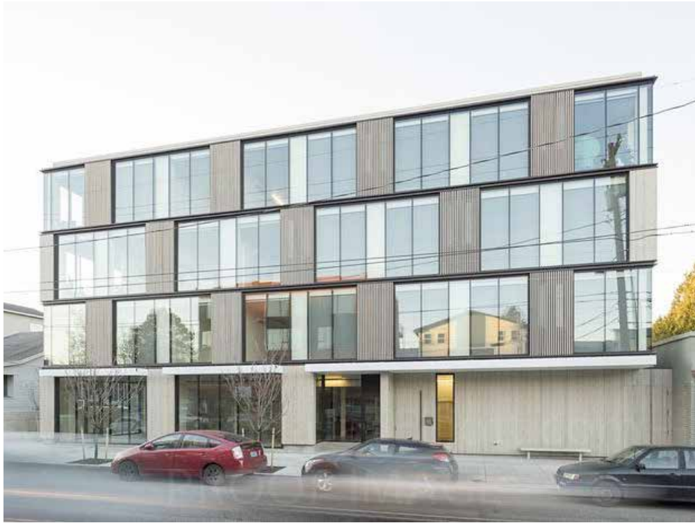
ANGLED PLANES WITHIN WINDOW BAYS
