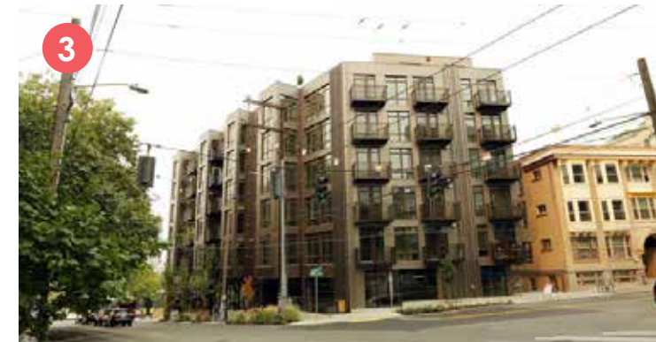
3 BROADCAST APARTMENTS • UNIFIED MATERIAL/FINISH, STRONG BAY EXPRESSION, • FULL HEIGHT VERTICAL BANDING
