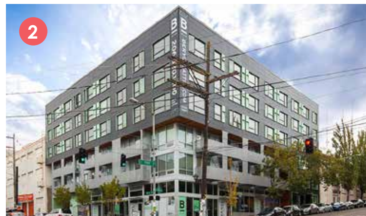
• TAUGHT SKIN SYSTEM, PAINTED METAL FACADE • DISTINCT RETAIL BASE
