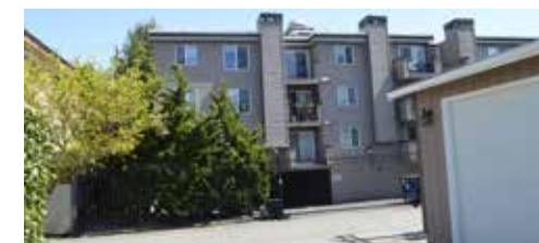
9. LOOKING E @ EX. CONDOMINIUM
