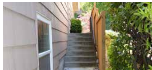
5. LOOKING WEST @ NORTH P.L.
