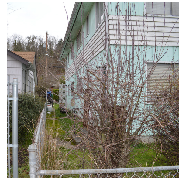
4. PARCEL A, SOUTHWEST PROPERTY CORNER
