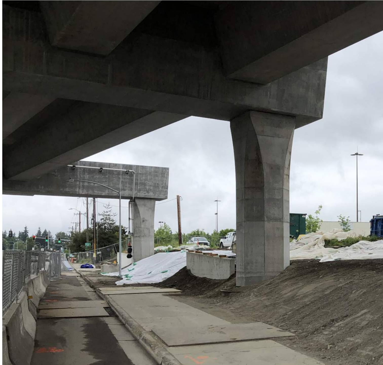
Existing Walls Along 1st Avenue NE
