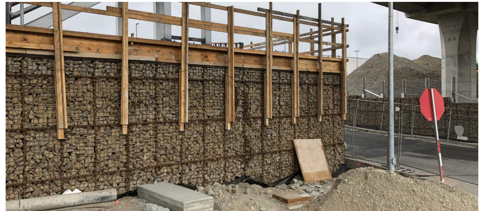
Gabion Wall Exposed at Corner of 1st Avenue NE and 105th
