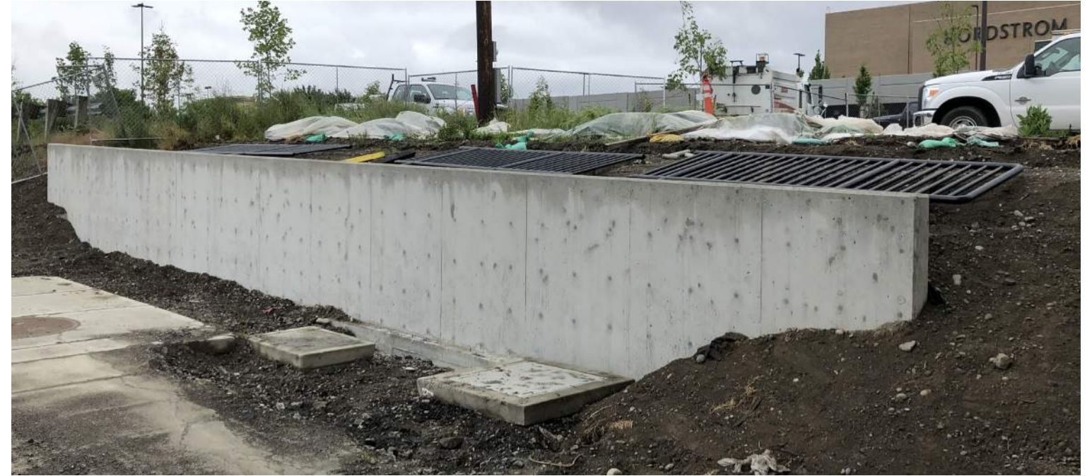
Concrete Walls Along 1st Avenue NE
