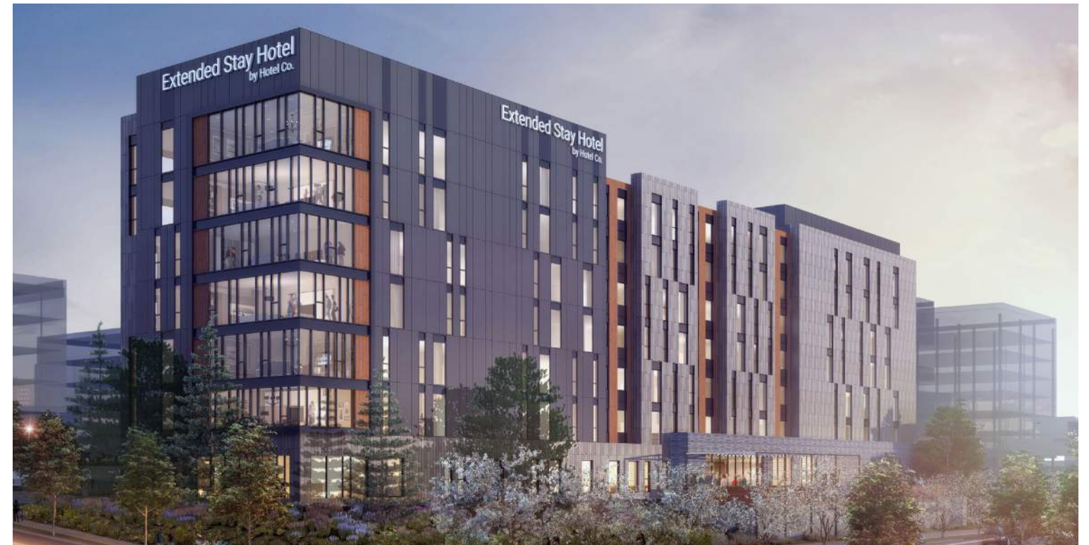
Previous NW Corner looking SE
