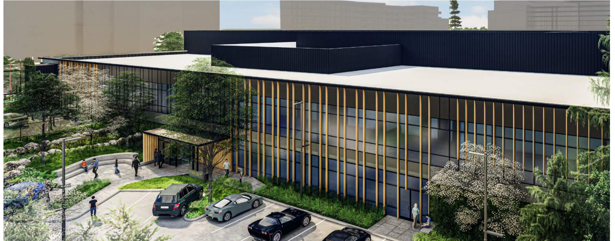
DRB 1 - Aerial Roof View
