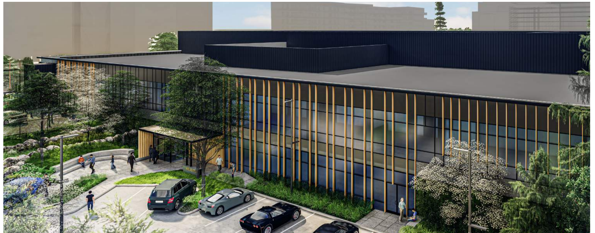
CURRENT - Aerial Roof View
