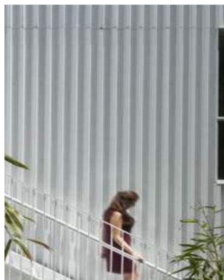
Random Mix or C-5 (4") / C-6 (8") Metal Wall Panels by Taylor Metal Products, 24 gauge in "Glacier White" and "Black"
