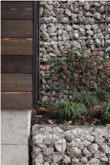
Integration of Gabion walls, concrete, cedar siding
