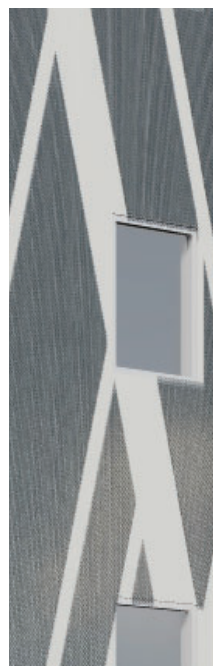
19 - PERFORATED METAL - FOCAL FEATURE WALL ALUMINUM NATURAL
