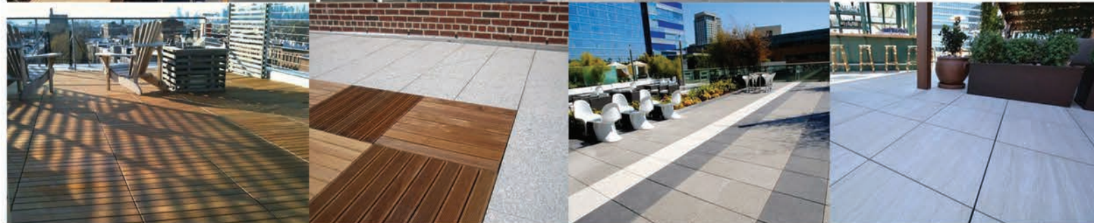
PAVING - WOOD - WOOD/CONCRETE - CONCRETE - PORCELAIN
