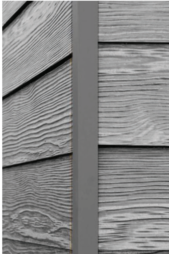
4 - HARDIE-PLANK FIBER CEMENT 6" LAPPED SIDING WOODTONE STAINED: CASCADE SLATE METAL OUTSIDE CORNER TRIM
