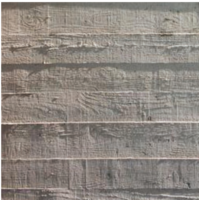
1 - BOARD FORMED CONCRETE COLOR: NATURAL / HORIZONTAL
