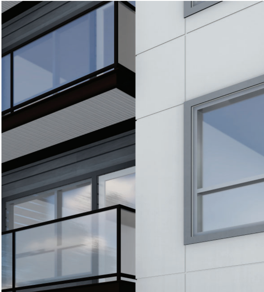
5 - HARDIE-PANEL FIBER CEMENT (5/16") PAINTED W/ REVEALS COLOR: SHERWIN-WILLIAMS PURE WHITE SW 7005 10 - VINYL WINDOWS WITH TRIM COLOR: WHITE TRIM: WOODTONE CASCADE SLATE
