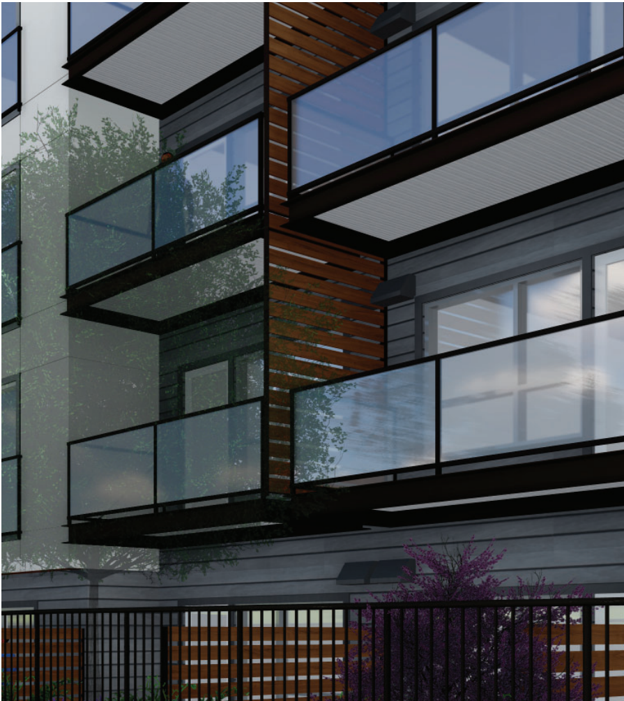
22 - PRIVACY SCREENS (SEE ABOVE) 16 - GLASS BALCONY RAILING / DARK BRONZE FRAME 17 - BALCONY - METAL FABRICATION DARK BRONZE W/ ALUMINUM PLANK 24 - VERTICAL PICKET ALUMINUM FENCING AND RAILING COLOR: DARK BRONZE
