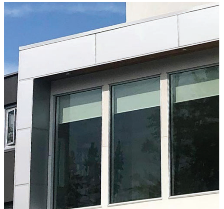
21 - 4MM ALUMINUM COMPOSITE PANEL COLOR: WHITE - FRAME - SOFFIT @ COMMERCIAL FRONTAGE - INSET WALLS @ COURTYARD
