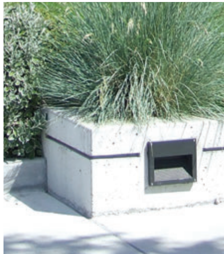
1 CIP WALL REVEAL + LIGHTS
