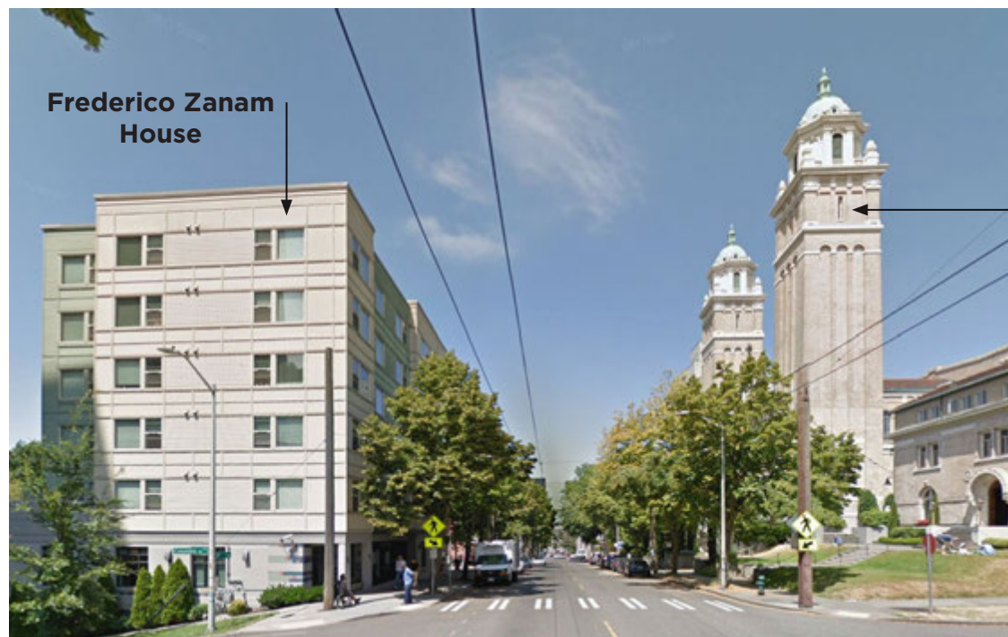
VIEW FROM 9th AND COLUMBIA LOOKING NORTH
