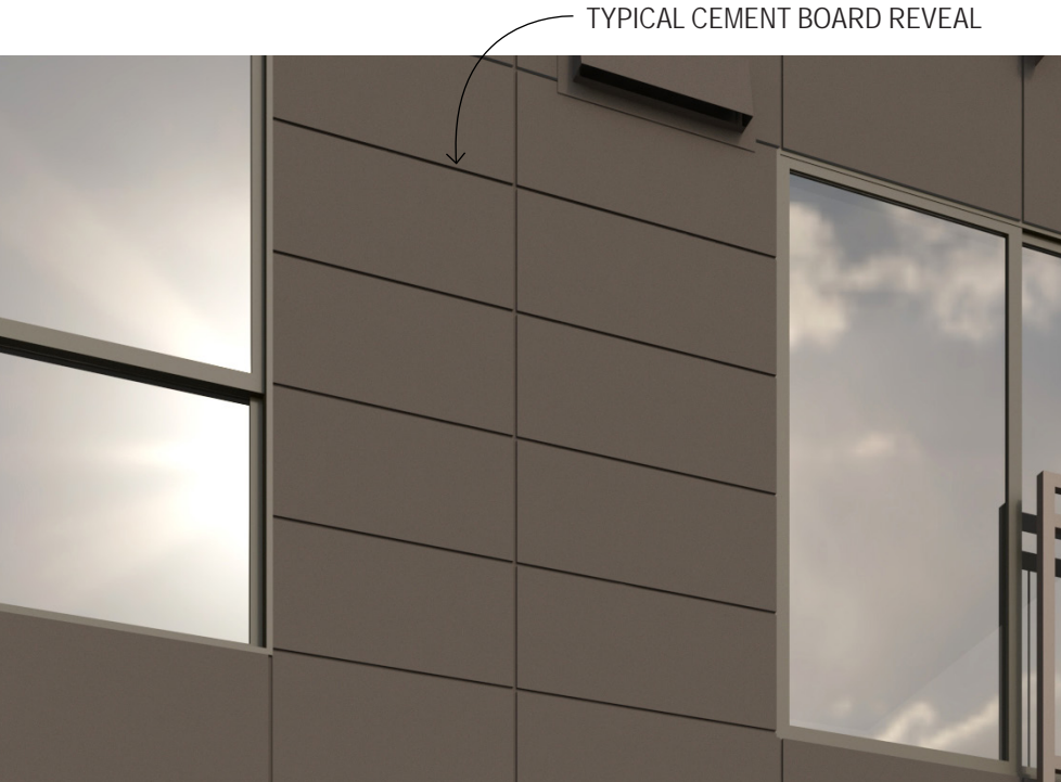
TYPICAL CEMENT BOARD PANEL REVEALS
