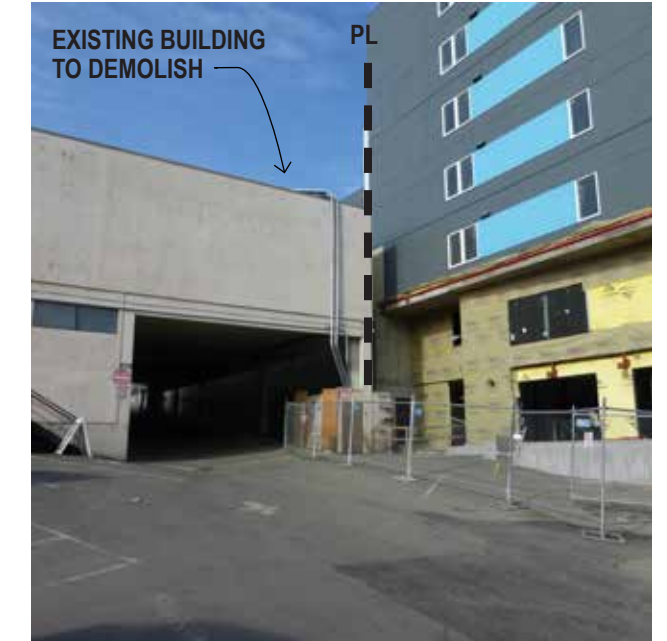
J EASEMENT LOOKING WEST
