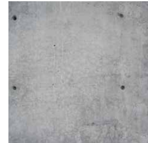
EXPOSED CONCRETE - AT EASEMENT
