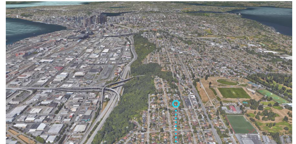
3626 AERIAL VIEW NORTH
