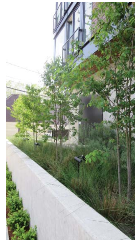
bioretention planter w/trees
