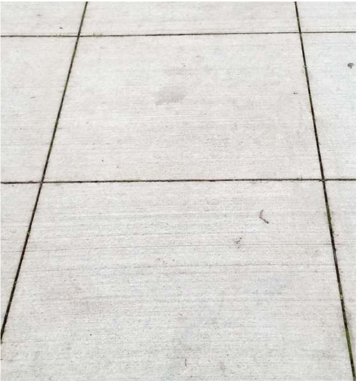
STANDARD GRAY SAWCUT SIDEWALK
