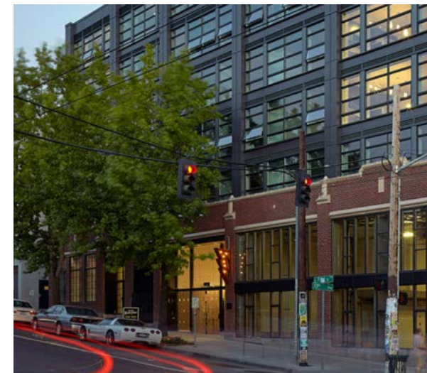
Traditional masonry massing and fenestration using contemporary materials.
