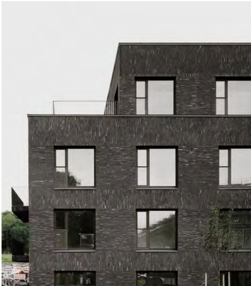
LARGE WINDOWS SET IN BRICK VENEER
