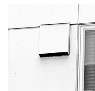
⑬ FORMED SHEET METAL VENT EXHAUST Sheet metal vent shroud, painted to match adjacent siding color
