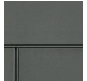
⑫ BLACK PAINTED HARDIE PANEL Countersink and fill fasteners, painted seams
