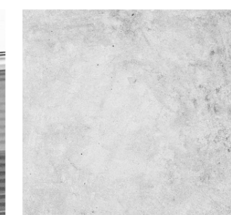
⑭ CAST-IN-PLACE CONCRETE Smooth form finish
