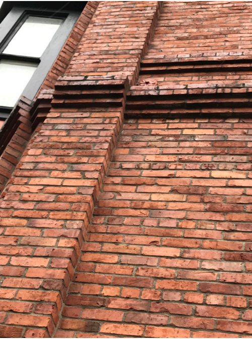
03. LOUISA BUILDING BRICK BANDING DETAIL AT FLOOR LEVELS
