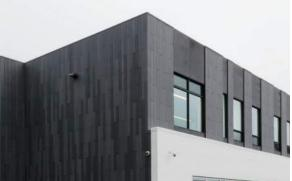
VERTICALLY ORIENTED FIBER CEMENT SIDING
