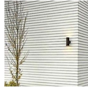
4" HORIZONTALLY ORIENTED LIGHT LAP SIDING
