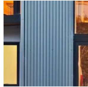
CORRUGATED METAL SIDING, VERTICALLY ORIENTED
