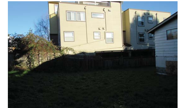
3 ADJACENT BUILDING TO NORTH
