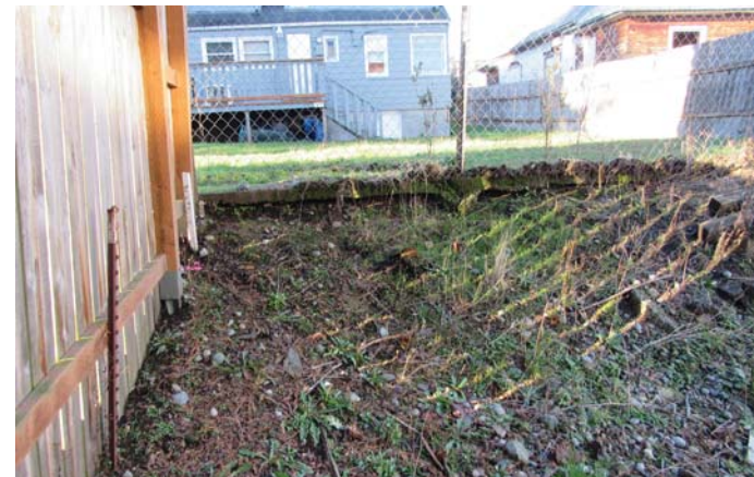
4 REAR YARD SOUTHWEST CORNER
