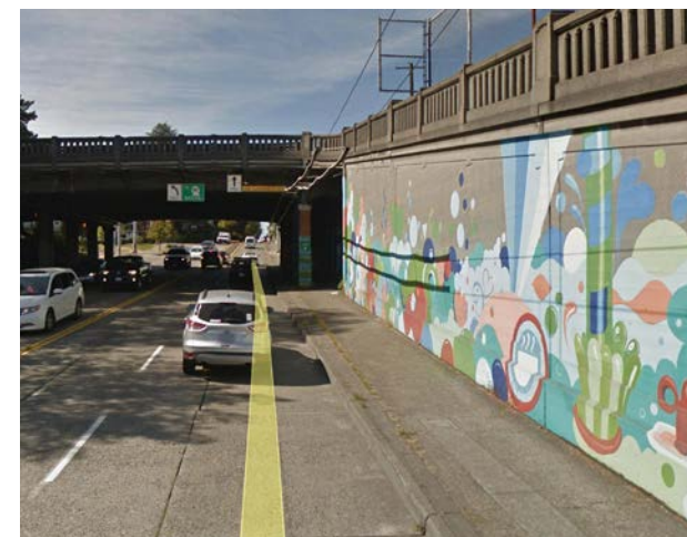
C. 46th St Underpass - access to transit
