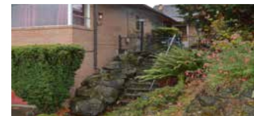
9. VIEW OF EXISTING DUPLEX
