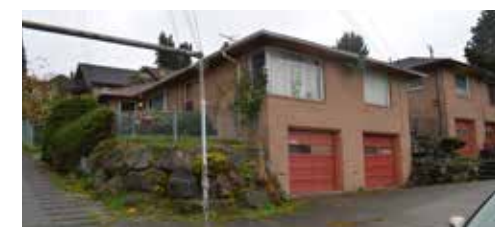
10. VIEW OF EXISTING DUPLEX
