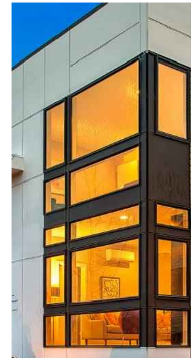
BLACK WINDOW TRIM ON WHITE HARDIE PANEL-SIDING
