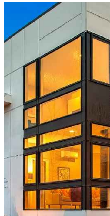
BLACK WINDOW TRIM ON WHITE HARDIE PANEL-SIDING
