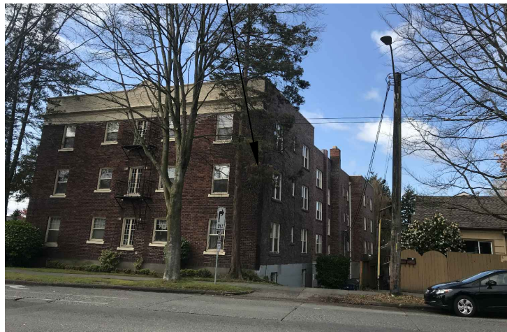
BEACON AVE SW FACING THE SITE (PROPOSED)
