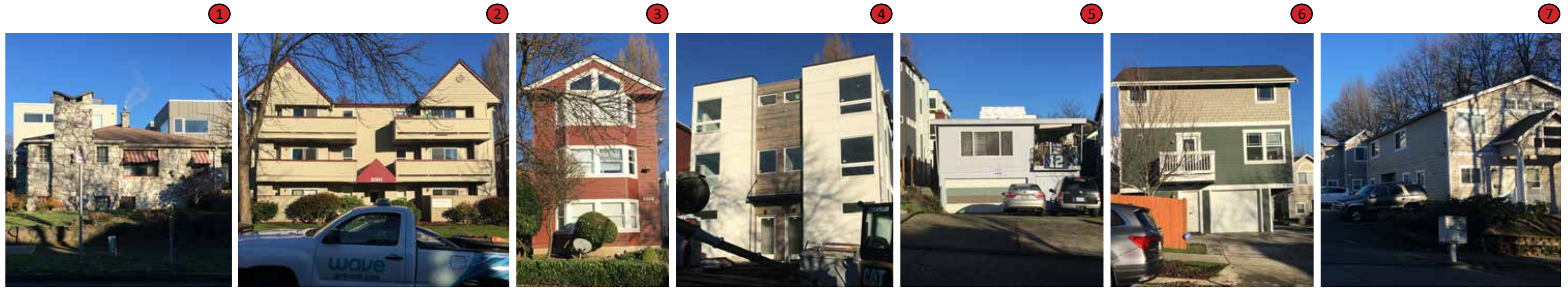
SOUTH MAIN STREET PANORAMA LOOKING NORTH
