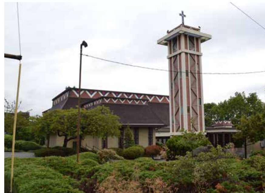
③ Mt Zion Baptist Church 1634 19th Ave Built: 1962
