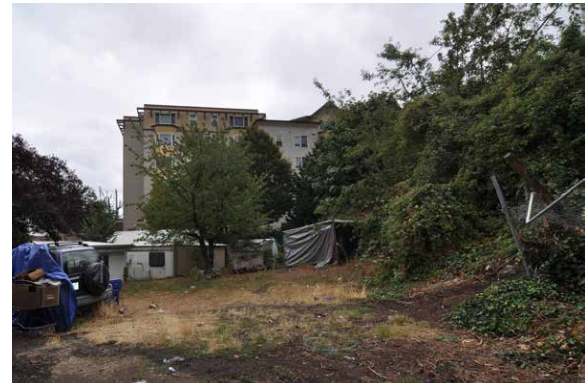
① View to Southeast property line condition
