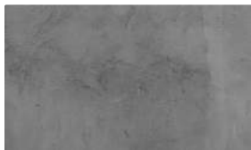
Concrete Foundation & Retaining Walls
