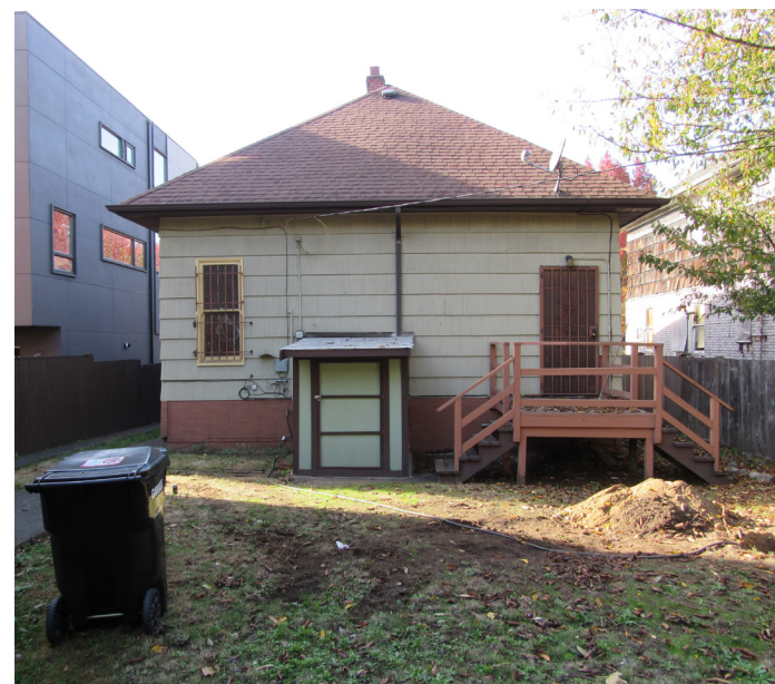
11 EXISTING BUILDING ON PROJECT SITE
