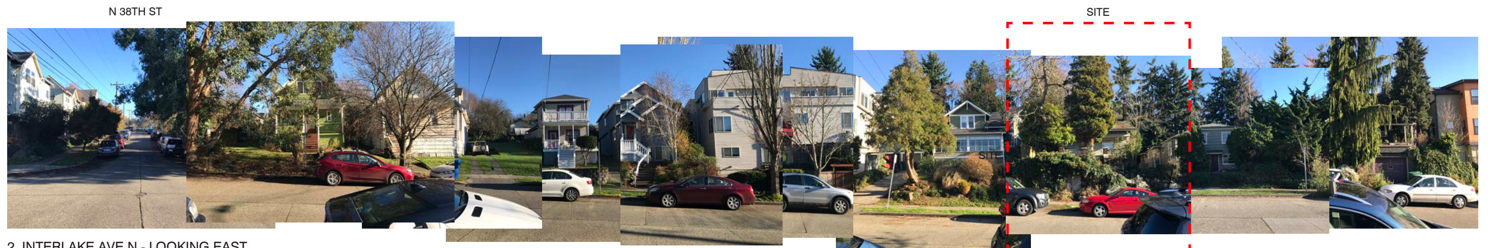
2. INTERLAKE AVE N - LOOKING EAST
