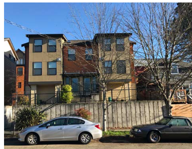
6. Townhouse Development South Of Site
