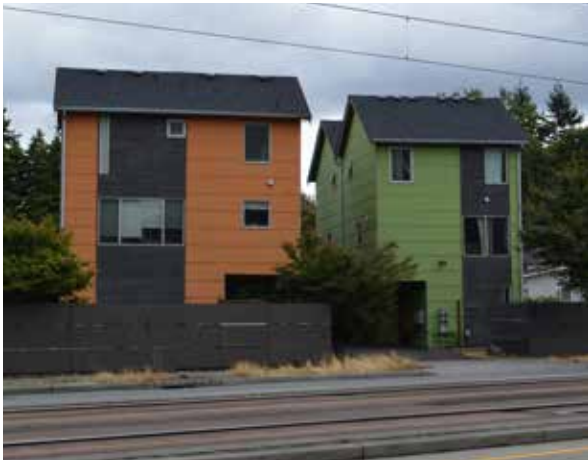
④ Townhomes 5036 MLK Way S Built: 2008, 5 units Street fronting setback with fence
