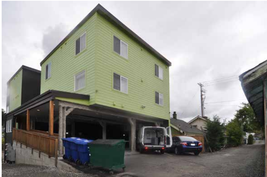
4 View of site looking Northwest from the Alley
