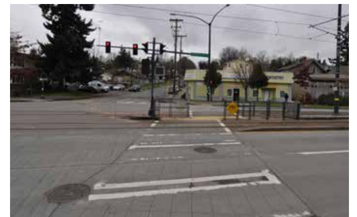
③ Crosswalk at Martin Luther King Jr Way S
