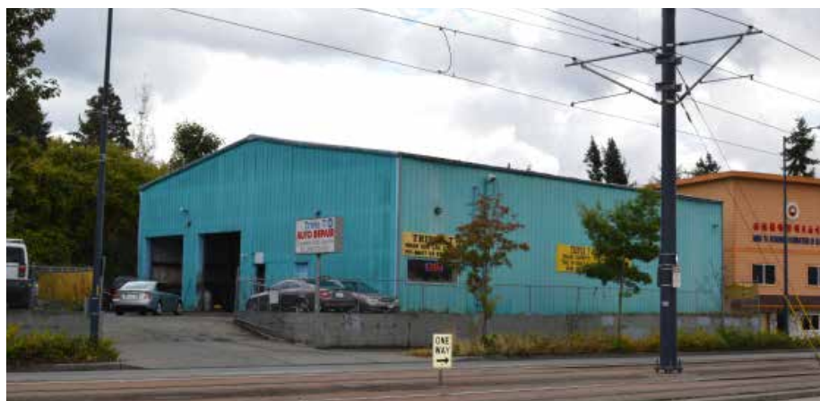
9 Service Building (Triple T Auto Repair) 5500 MLK Jr Way S Built: 2000 Blank wall along Martin Luther King Jr Way S
