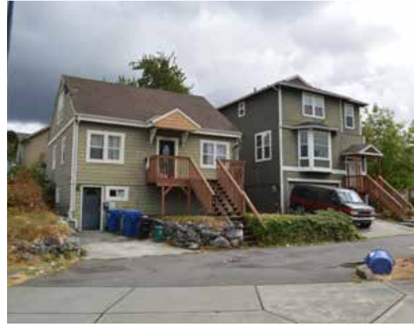
② Single Family Homes 5218/5222 35th Ave S Built: 1929, 2006 Elevated residential entries along Martin Luther King Jr Way S
