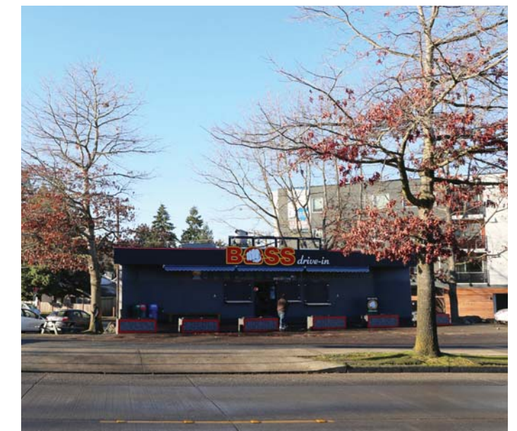
6 DELRIDGE WAY SW, LOOKING WEST
