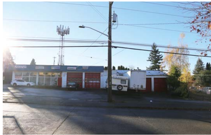
1 LOOKING SOUTH FROM SW BARTON ST.
