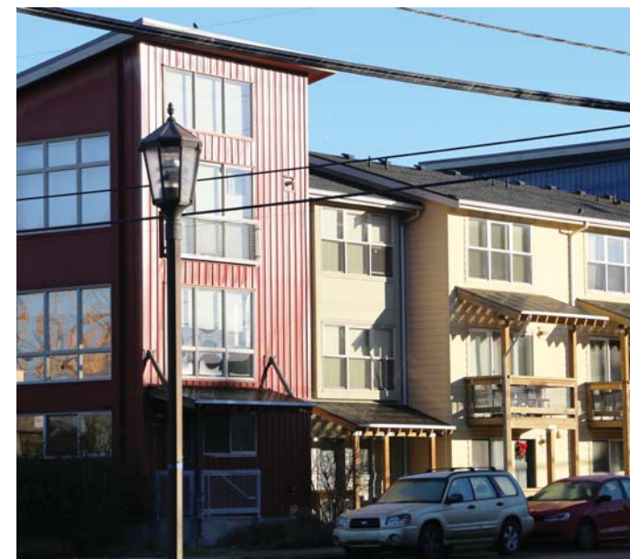
5 18TH AVE SW, LOOKING EAST
