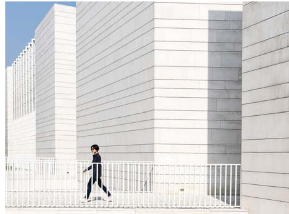
Monolithic facade interrupted by heavy recesses and access points.
