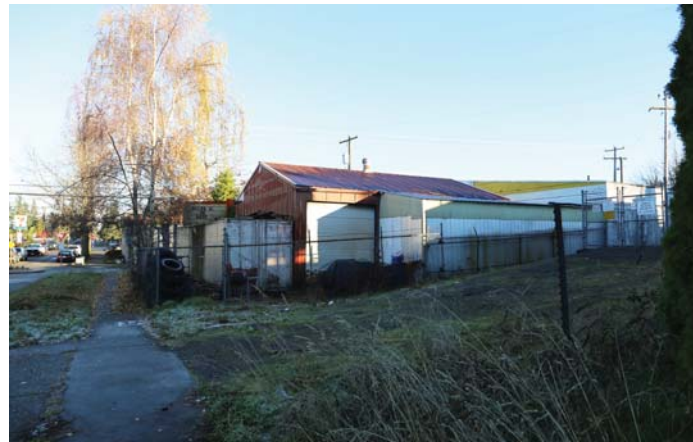
4 LOOKING NORTH ON 20TH AVE SW
