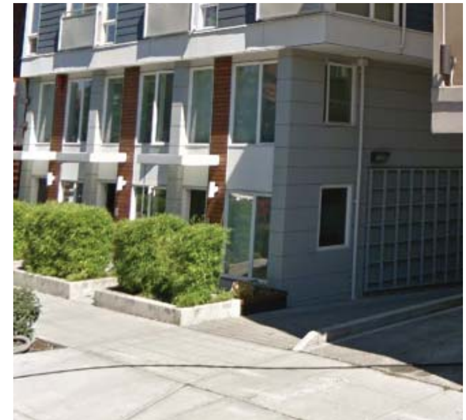
10' wide driveway accessed from Bellevue Avenue at the Local 418 apartments
