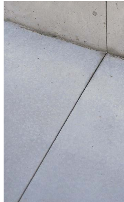
concrete with sawcut joints
