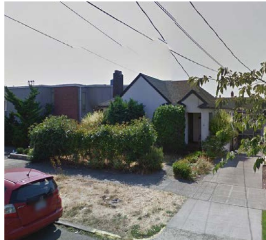
2 Existing Single Family House on Project Site
