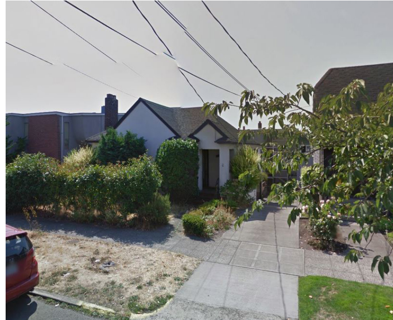
2. view of existing house on property / shared driveway easement
