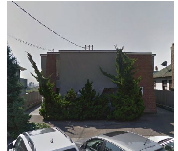
10 Adjacent Apartment building to the east of site
